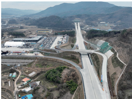
Pyeongtaek-Buyeo (Western Inland) Expressway Bongsusan Tunnel mechanical equipment
